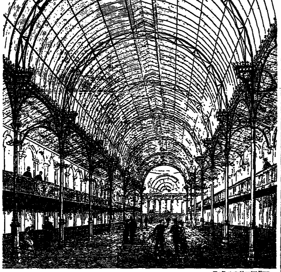
An 1887 impression of the interior of the Floral Hall, built in the style of the Crystal Palace. Right: market bustle early this century
